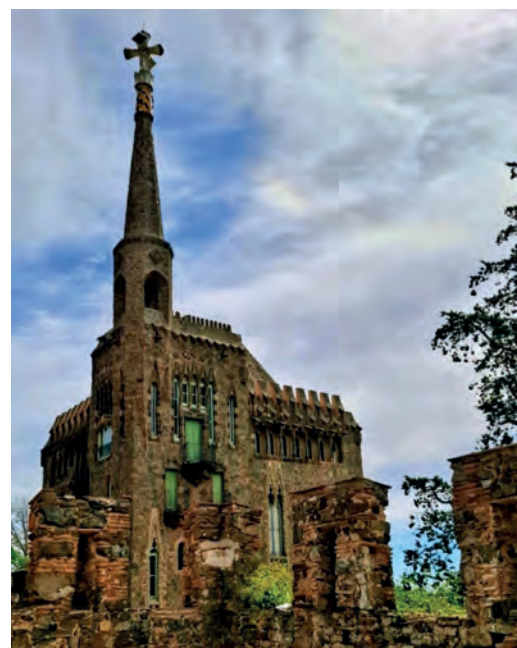
Torre Bellesguard, Barcelona
